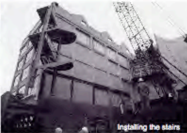
Installing the stairs
